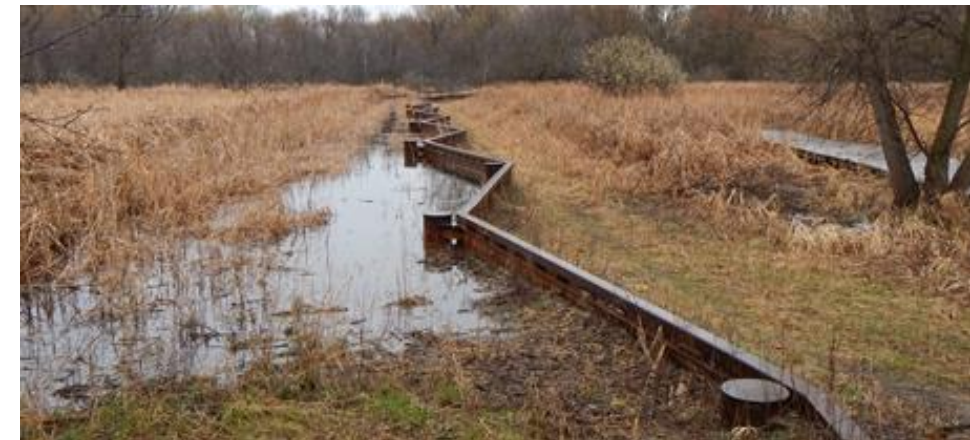
Photo: example of a sheet pile weir
