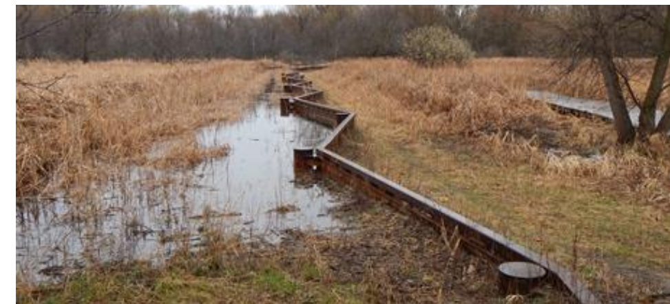
Photo: example of a sheet pile weir
