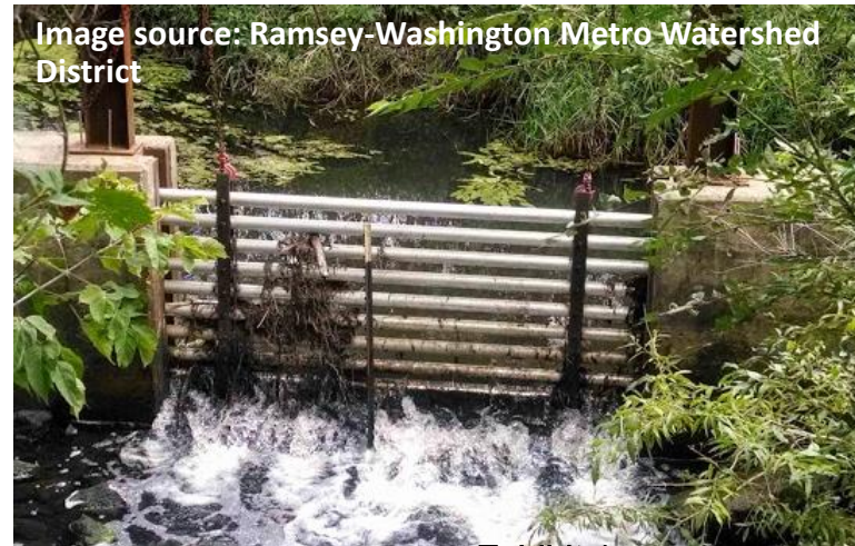
Exhibit 1 Photo: adjustable/sliding gate barrier
