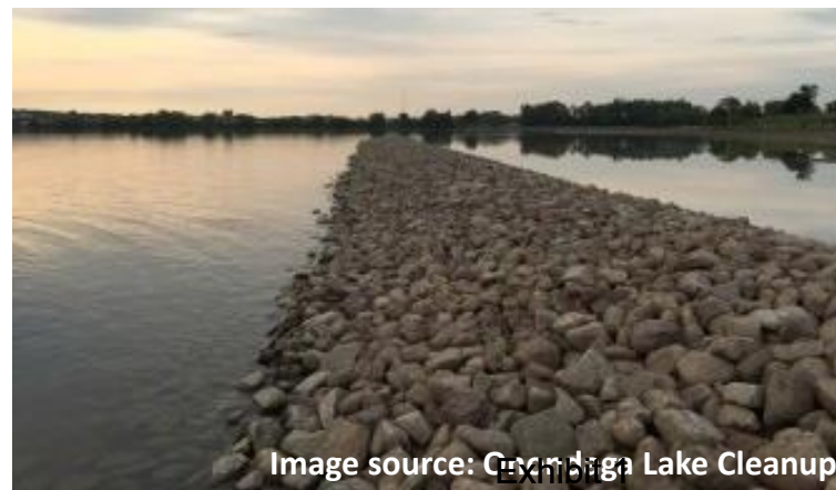
Photo: example of a rock berm
