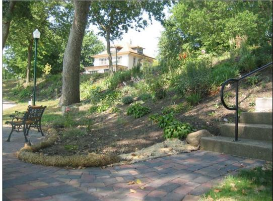
Plantings and a lake log to control erosion on a steep hillside in Fulda,
