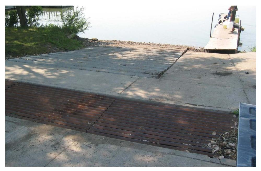
A grate on a boat ramp will prevent debris from entering Fulda Lake
